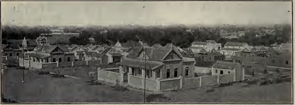
BLOCKS OF BUILDINGS UNDER CONSTRUCTION IN FRASER TOWN
